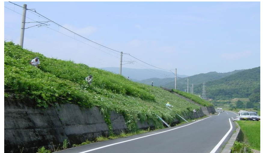
Glass cutting of slope of railroad 線路の法面清掃
